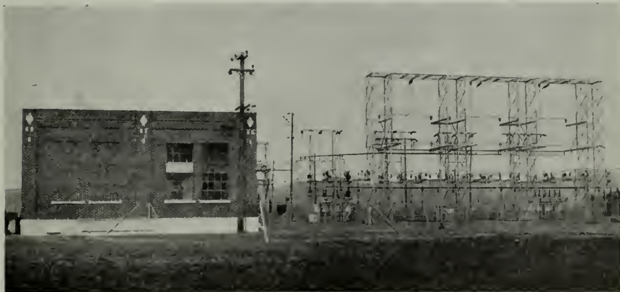
Union Gap Substation - constructed in 1930 by Pacific Power & Light Company.
